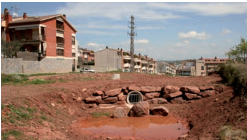
Soterrament Colector Ermots
